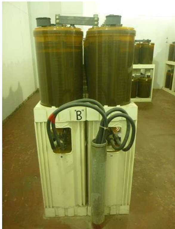
Station Service B – 60 1600AH ATT Round Cells – East Side of Room.
