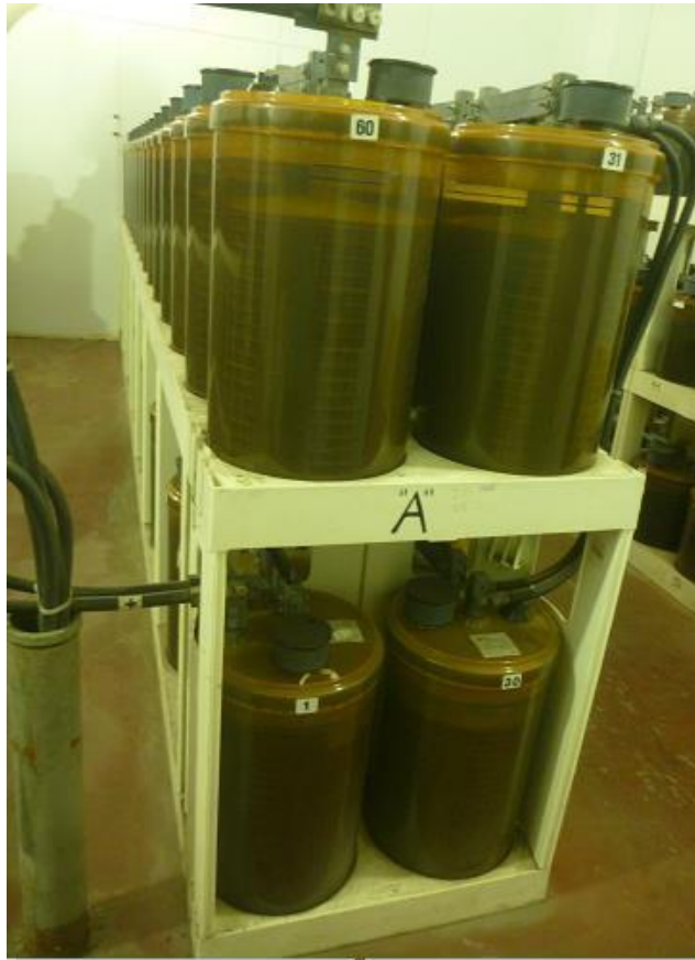
Station Service A – 60 1600AH ATT Round Cells – Center of Room.
